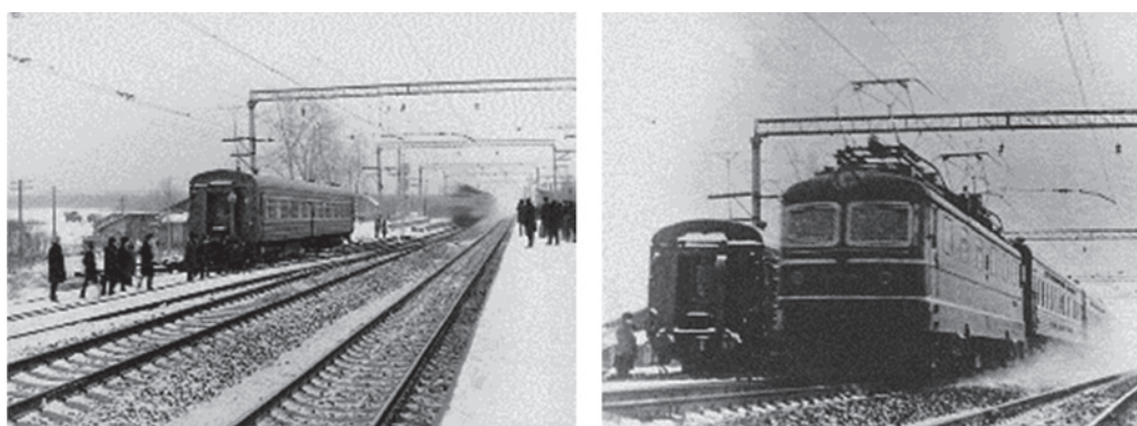
Fig. 8. Testing of a turnout designed by the Design Bureau of the Main Railway Department of the Ministry of Railways and Leningrad Institute of Railway Engineers (LIIZhT) with a movable frog core at Pomeranye station of Oktyabrskaya Railway. A train running at a speed of 228 km/h, 26 February 1971 [11]
