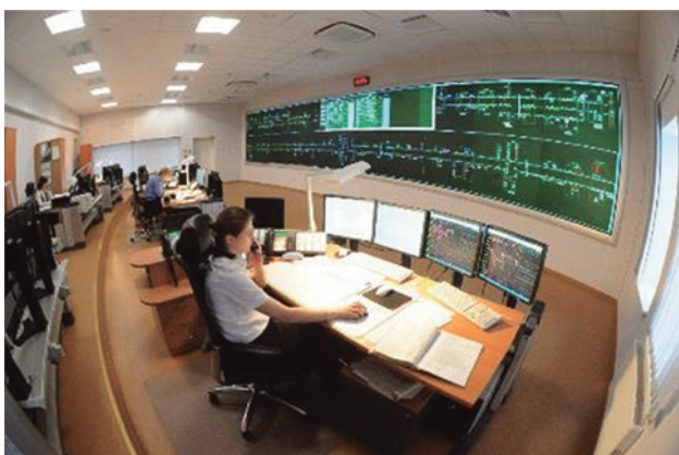
Fig. 14. Unified Dispatch Control Centre of Oktyabrskaya Railway, 2009. Photo by I. Kurtov
