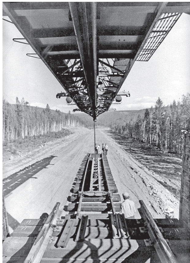
Track laying on the central section of the BAM. 1970s. (Science and Technology Library (NTB) of PGUPS)
