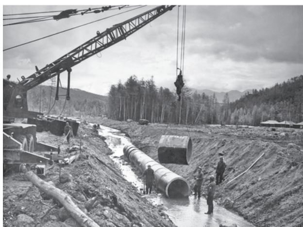
LIIZhT students building a drainage collector for the east portal of the Severomuysky Tunnel. The Buryat section of the BAM. 1977. (Photo by S.F. Spiridonov, collection of A.V. Kabanov. Science and Technology Library. PGUPS)
