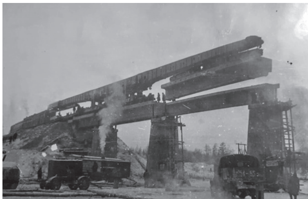
Military railway workers are replacing temporary spans with permanent ones on the river between 70 km and 90 km from Tynda. Early 1980s. (Photo from the collection of N.S. Rogalev. Science and Technology Library (NTB) of PGUPS)
