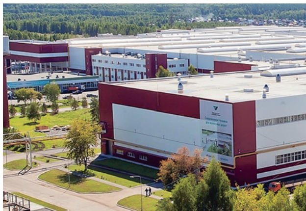
Fig. 20. General view of the production buildings of the Ural Locomotives Plant 2
