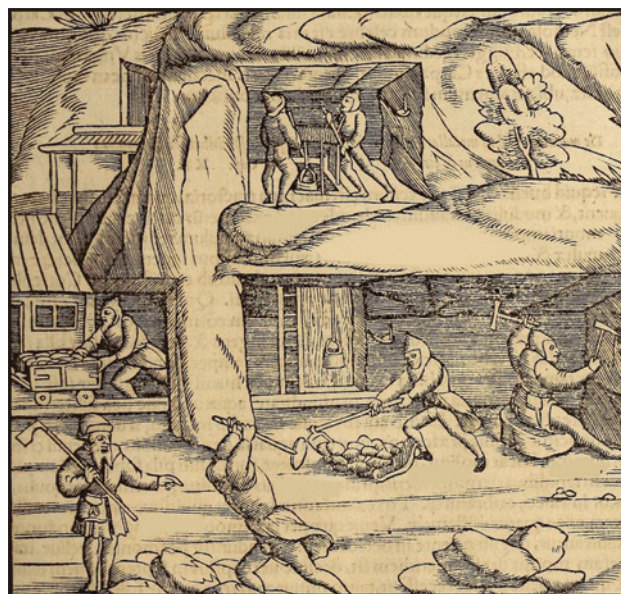
Fig. 1. Drawing of a mine road with a trolley, considered to be the first published drawing. 16th century. Fragment of an engraving. Universal Cosmography (Latin: Cosmographia universalis, 1544), a book by Sebastian Münster (1488–1552) [1]
