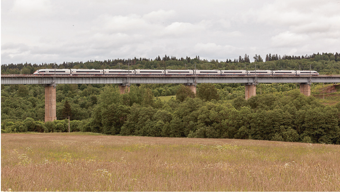
Fig. 10. New Verebyinsky Bridge with a running Sapsan train. 2001. Photo by Mikhail Krivykh 12
