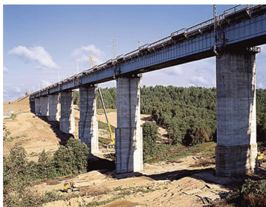
Fig. 9. Construction of the new Verebyinsky Bridge. 2001. Photo by Mikhail Krivykh 11
