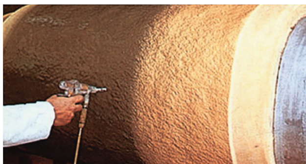
Fig. 7. Application of thermal insulation from rigid polyurethane foam [23]
