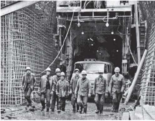
Members of a LIIZhT student construction brigade at the construction site of the Severomuysky Tunnel on the BAM. Late 1970s. (Photo by PGUPS)
