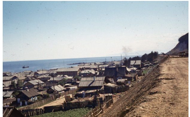
Roadbed of the future line. 1980. (Photo by E. Komarov. Science and Technology Library (NTB) of PGUPS)
