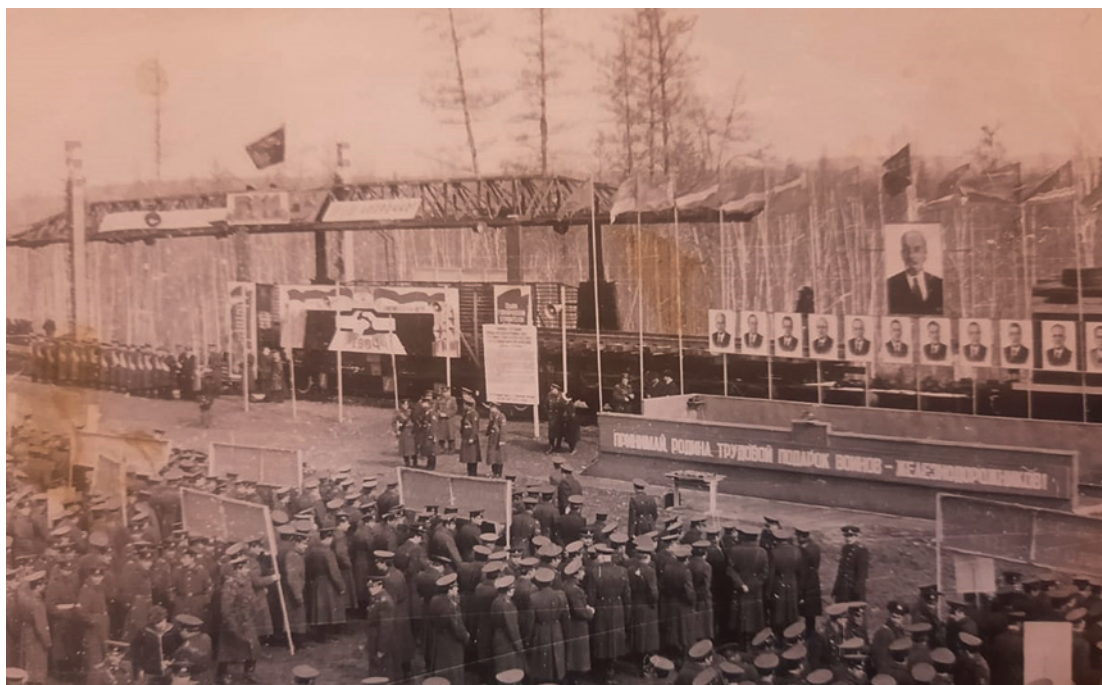
Miroshnichenko junction, 497 km. Military railway workers are laying the final rail length with the golden spike on the Tynda–Urgal section during a ceremony dedicated to the occasion. April 17, 1984. To provide the possibility of through traffic, the sections of the 35th Railway Corps (also known as the Tynda Corps) and the 1st Railway Corps (Urgal Corps) were connected to produce a total length of about 1,000 km and open through traffic. (Photo from the collection of N.S. Rogalev. Science and Technology Library (NTB) of PGUPS). The “Golden Word” about military labour valour, responsible attitudes, and the sense of duty during the construction of the Baikal-Amur Mainline (URL: https://dzen.ru/a/Y3byG_R-fXGUjEyg )
