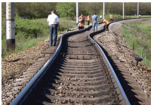
Fig. 1. Typical view of a bucked track section
